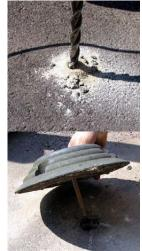
3. Clean hole of debris. Insert bolt shield into hole. Ensure you insert to a depth that the bolt can still screw into the nut.
